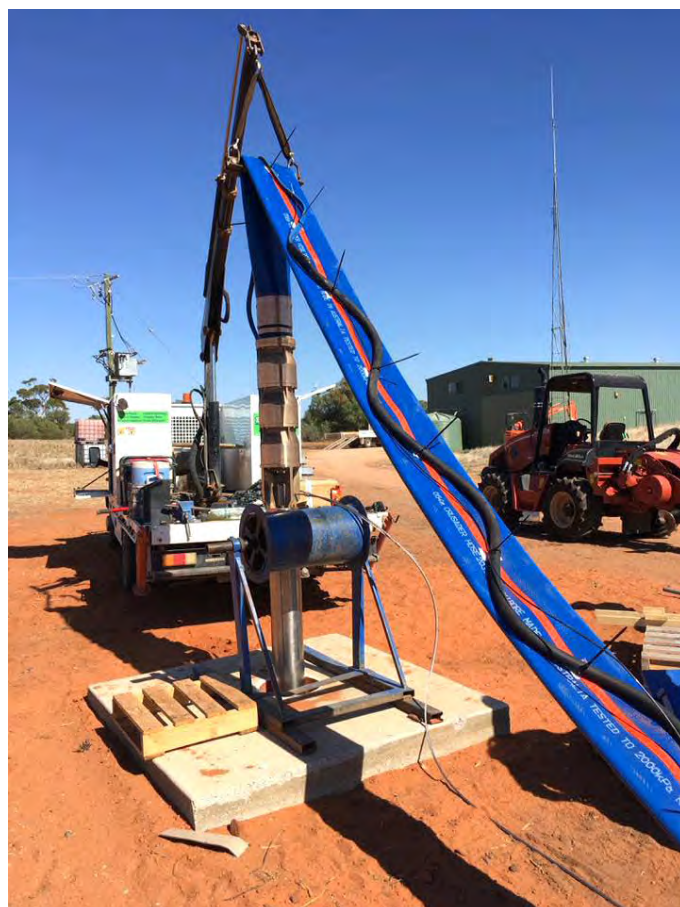
Submersible pumps that needed heavy-lifting equipment and days of work can now be installed and running within a morning.
