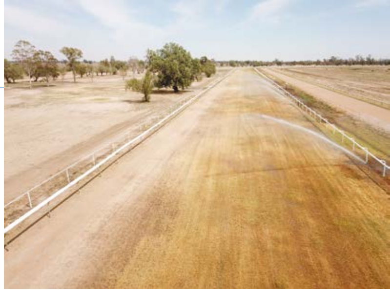
Coonamble Racetrack received its first application of water directly after the system was completed in December 2019.
