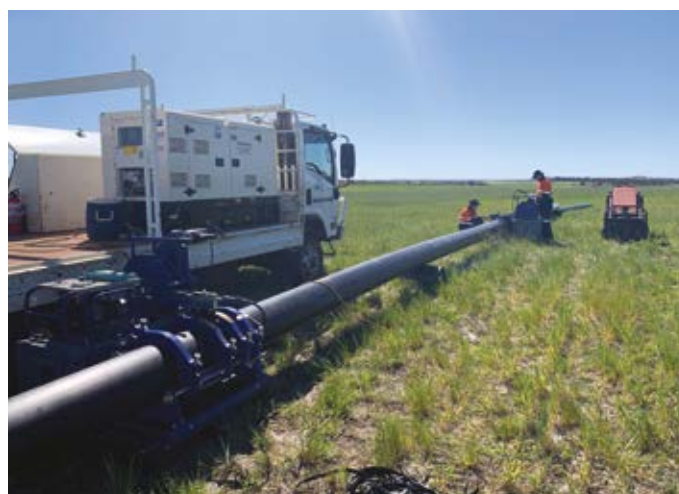
Staff from Watertorque Broome butt-welding a pipeline from a bore field made up of three 37 kW bores. The pipeline supplies a 24 ML storage with a 120 L/sec pump station, which then supplies water to a cattle feedlot.
