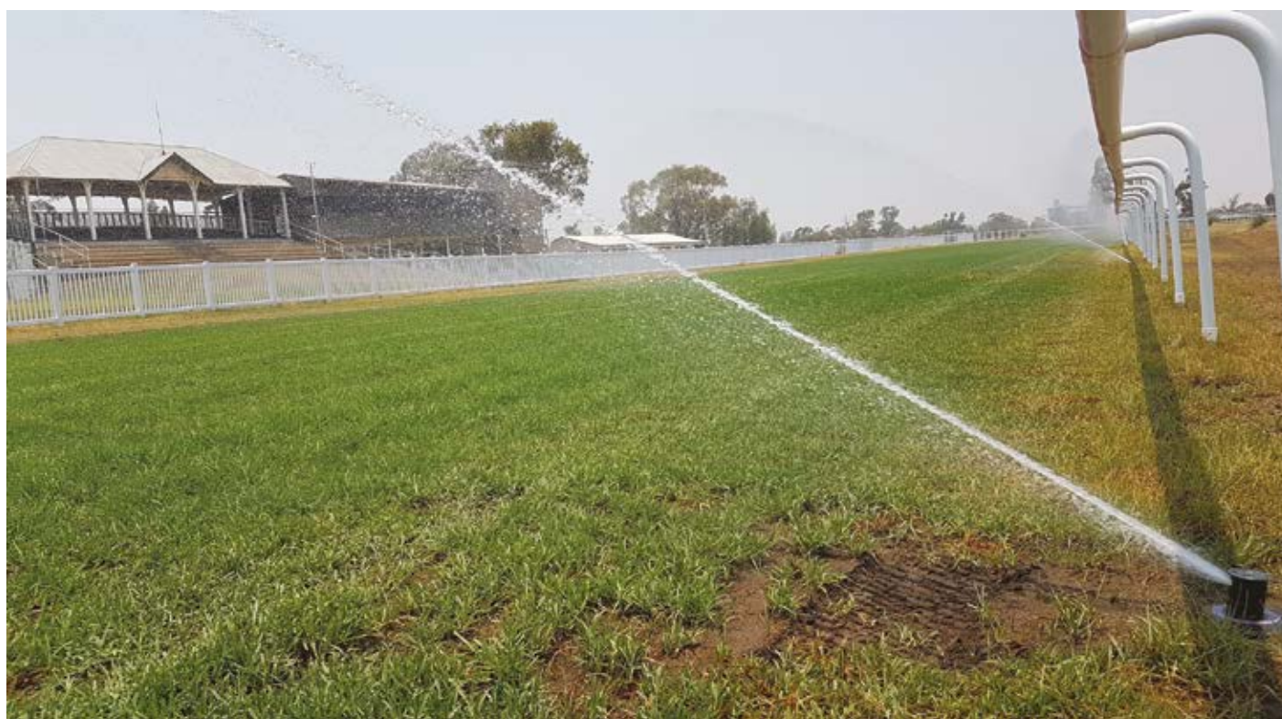
Placing the rotors to avoid horses hitting them and water being displaced by rails is an important consideration in design.
