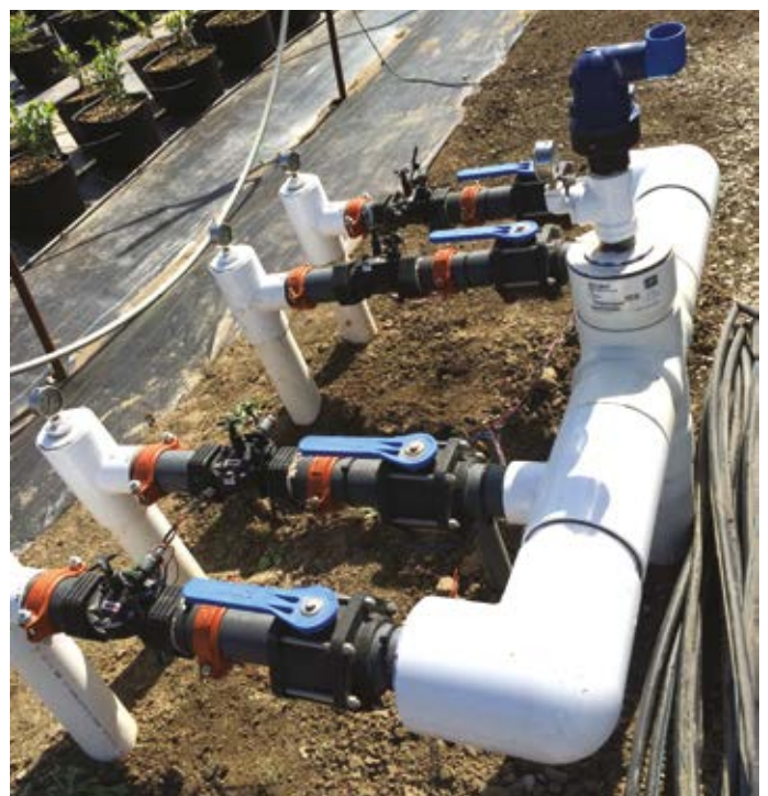
Above: This pump and filter station has two sustaining valves that help keep backpressure on the filters while irrigating strawberry fields below. Below: This electric throttling valve manifold allows the grower to control flow to four separate blocks and irrigate them individually or simultaneously.
