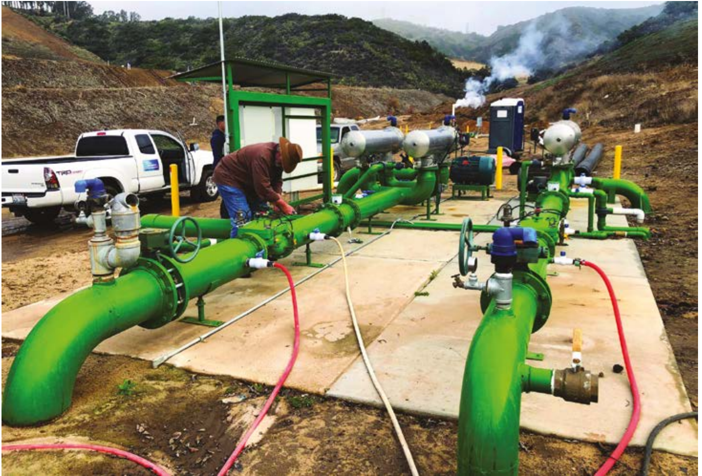
Above: This pump and filter station has two sustaining valves that help keep backpressure on the filters while irrigating strawberry fields below. Below: This electric throttling valve manifold allows the grower to control flow to four separate blocks and irrigate them individually or simultaneously.
