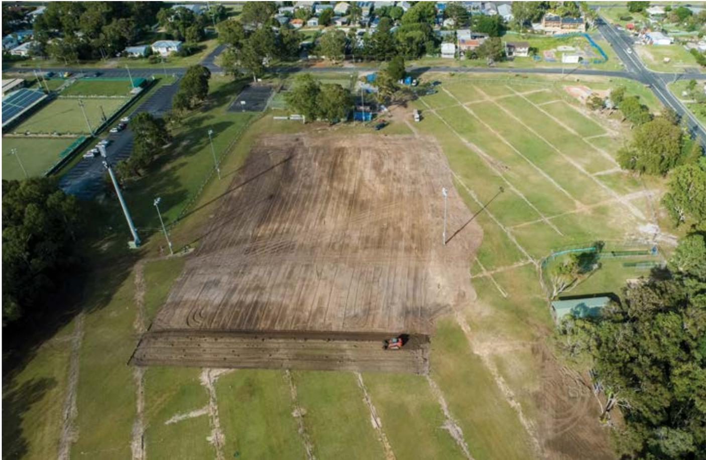
This overhead photo shows the oval during installation of irrigation infrastructure, as well as oval surrounds. The machine is using laser levelling to cut and fill the surface of the oval. The pipes and risers are already installed.
